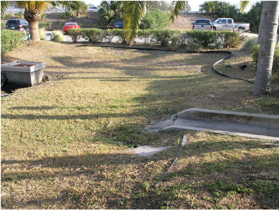
Figure 2. Greenspace area within a parking lot used for stormwater detention and infiltration.
