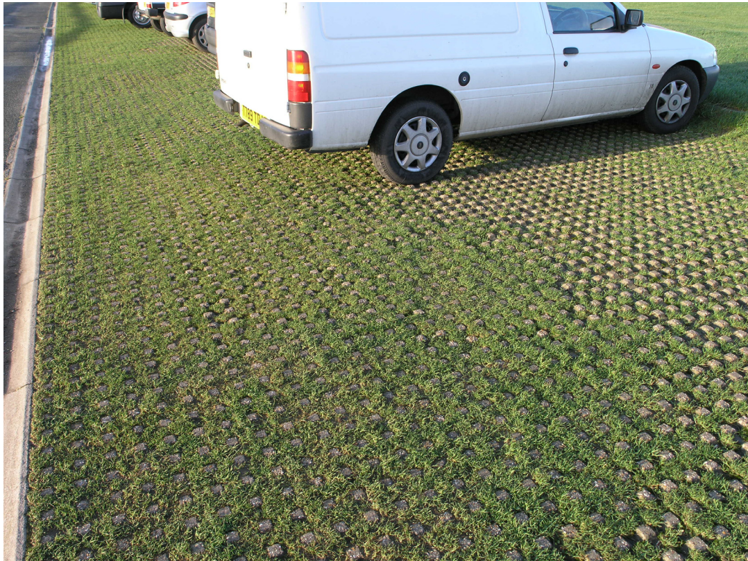
Figure 3. Perforated pavers used for parking spaces and stormwater infiltration.
